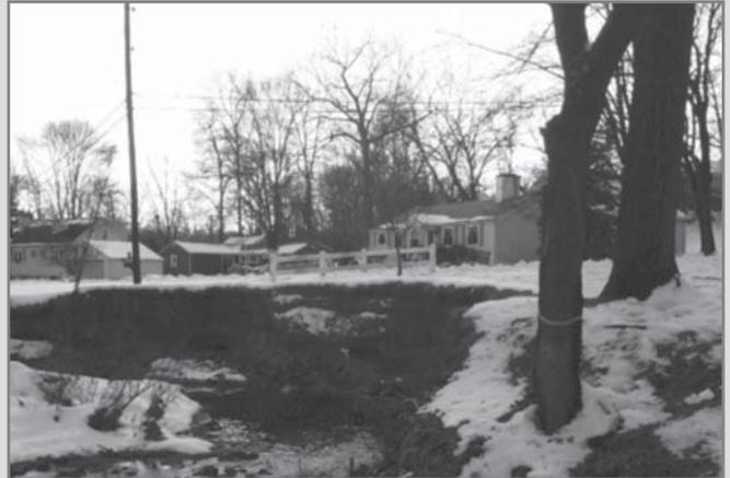
**PHOTO 1:** View of severely eroded bank prior to pre-bid meeting. (credit Rich Krasselt, BCCD)
