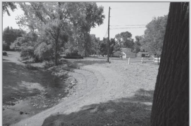
**PHOTO 3:** Stabilized bank 2 days following completion of construction.
