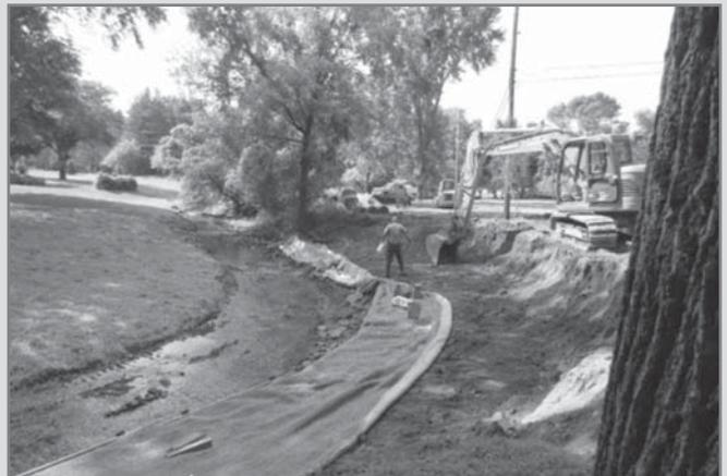
**PHOTO 2:** Dale Bentz of RiverLogic Solutions seeds the lowest soil lifts before fabric is staked in place.
