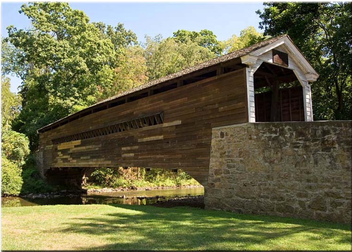
Rapps Bridge (Rapps Dam Rd, Phoenixville)
