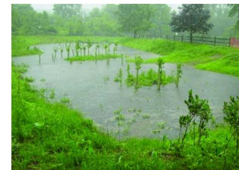
The basin operated as designed during this storm event on June 26, 2006. The created berms are evident as the basin fills.
