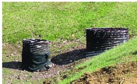
The modification to the outlet included covering the lowest opening with a geotextile and soil to create a shallow pool of water immediately after storm events.
