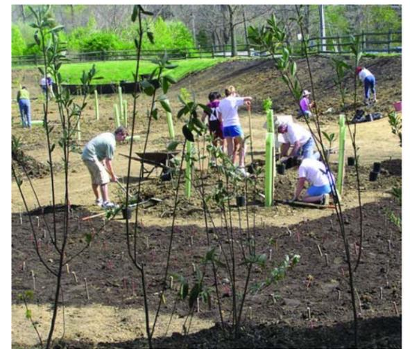
*The retrofit of this stormwater basin at Sidley Road included small berms to increase the length of flow to allow more pollutant removal, and planting over 400 trees and 300 live stakes in the 3/4 acre stormwater basin.*
