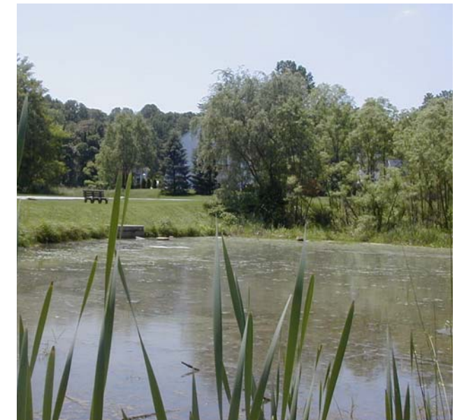
Stormwater retention basin (pond) integrates access for pedestrians as well as providing vegetation along the shoreline.
